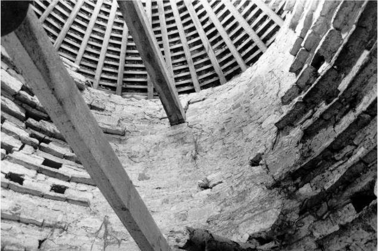
9 – Internal view showing rebuilt walling
