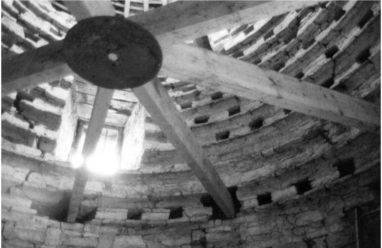
7. Modern inserted floor timbers
