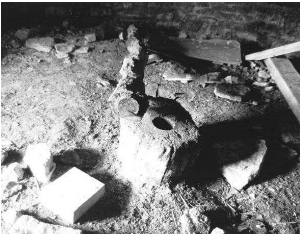
14 Central timber block and detached post
